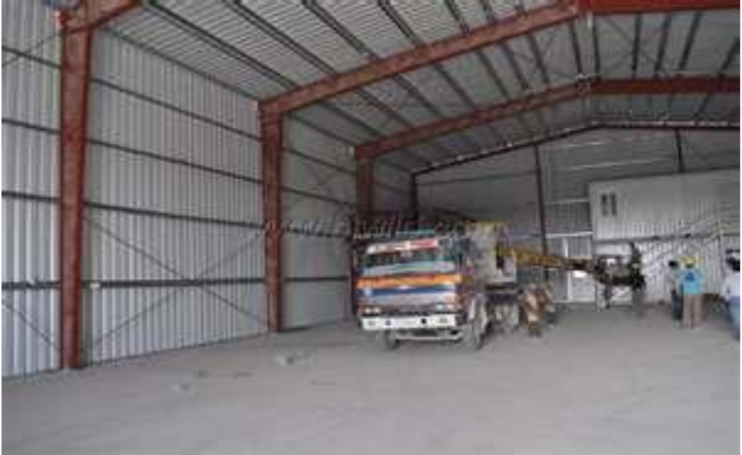
Steel frame with metal exterior walls
