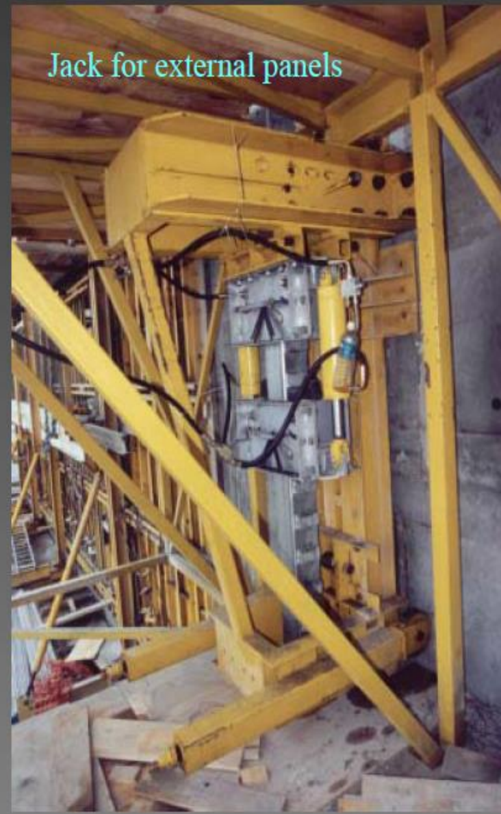
Close up view of the hydraulic jack
