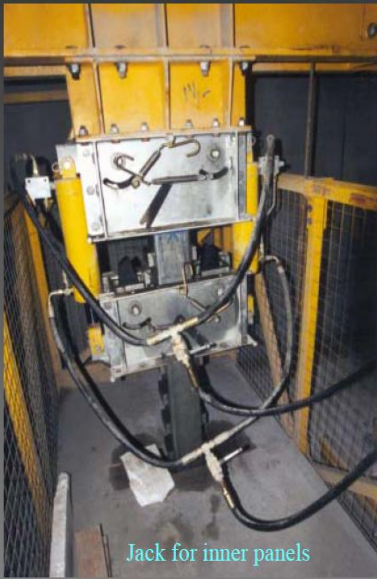
Close up view of the hydraulic jack
