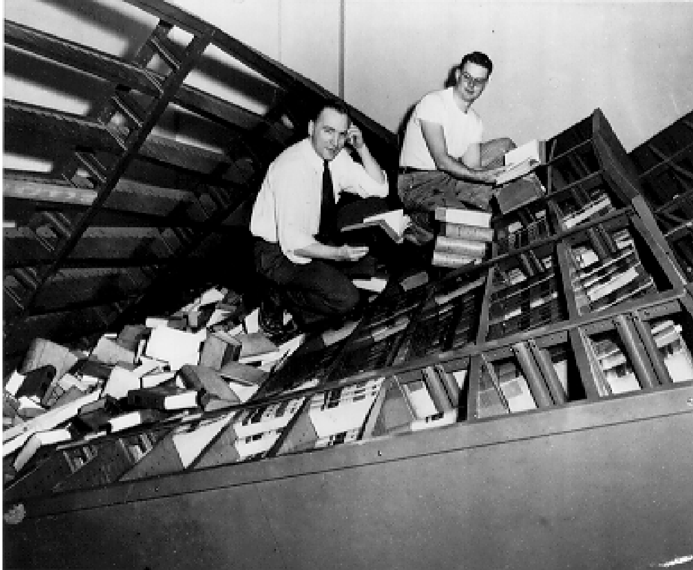
Library shelves overturned as a result of the 1949 Olympia earthquake. (Photo by permission of the Seattle Times Co.)
