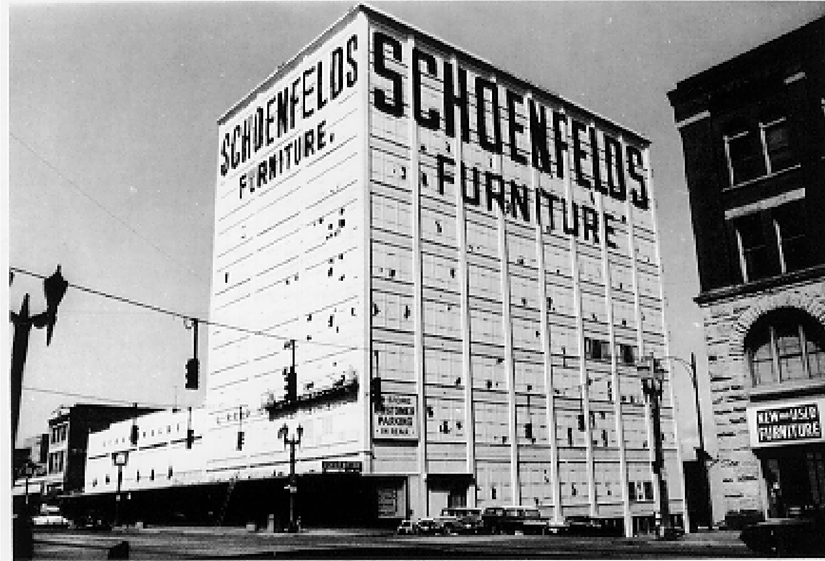
Glass windows broke on three sides of this ten-story building in Tacoma during the 1965 Seattle-Tacoma earthquake. (Photo by B. J. Morrill, from Steinbrugge and Cloud, 1965)
